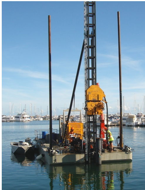
Piling Barge - Dunnit
