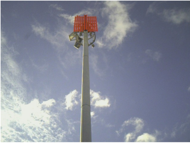
Inner Harbour Entrance Front
