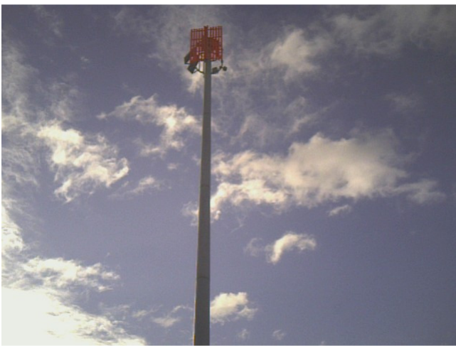
Inner Harbour Entrance Rear
